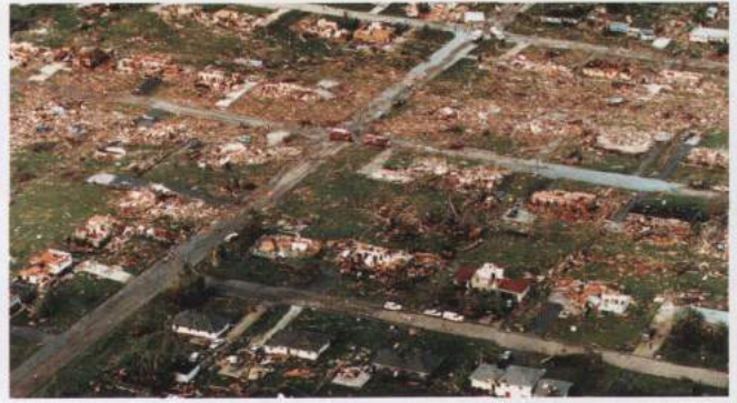
Severe damage shows the path of a tornado.
