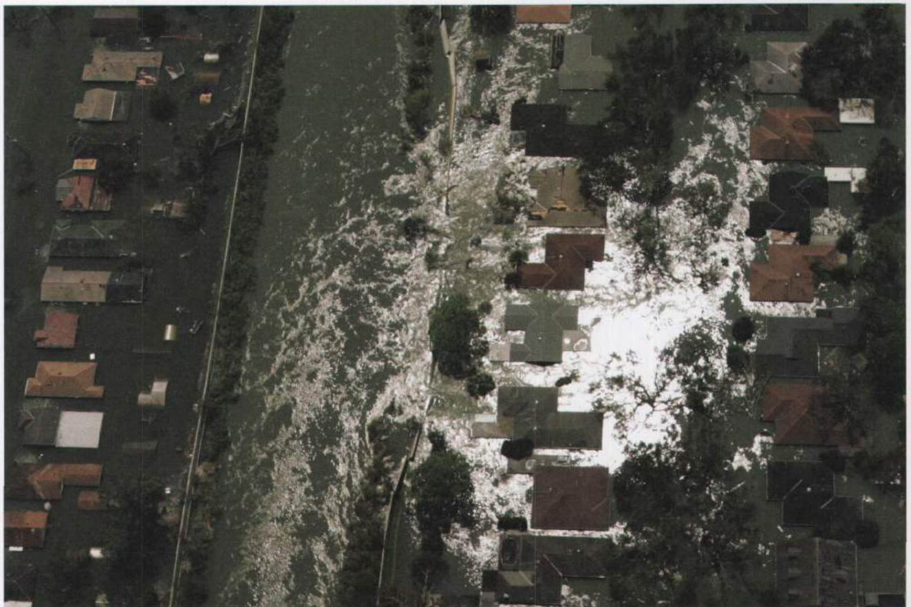
Floodwaters rush over the top of a levee into a New Orleans neighbourhood.
